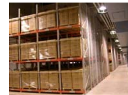
Warehouse for disaster supplies
