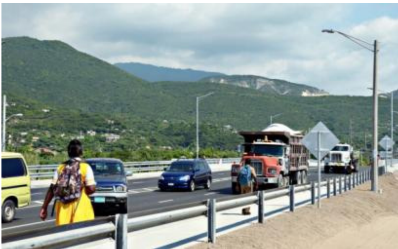
Plate 7: Post-construction phase of the bridge at Harbour View, St. Andrew. Source: OPM 2011.
