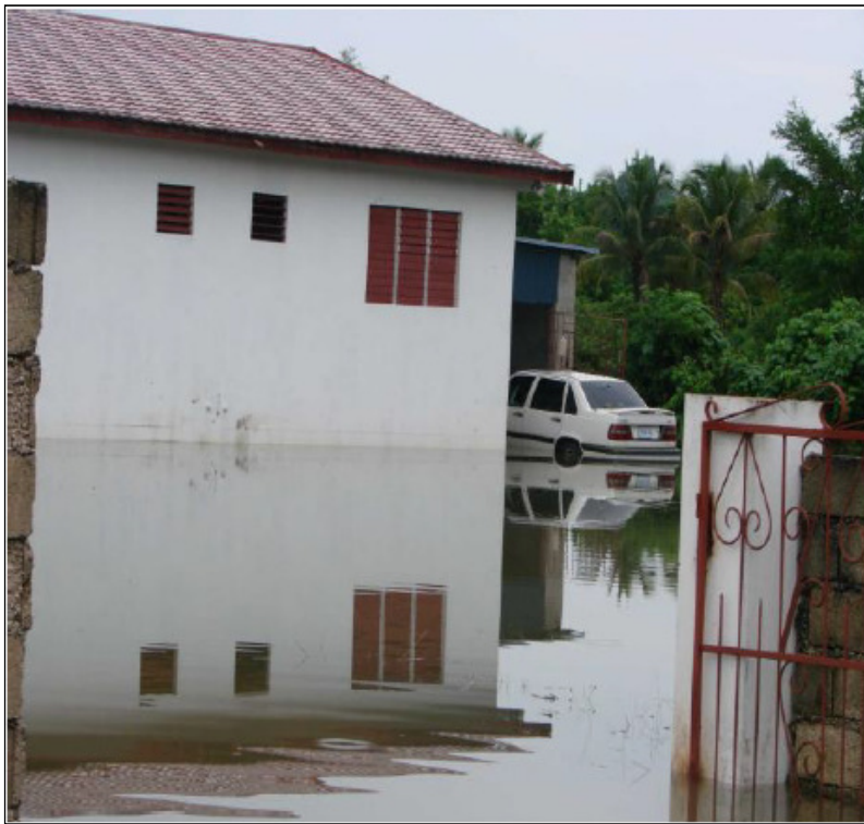
Plate 5: Inundated house in Wilton, St. Elizabeth in which senior citizens were trapped for four days after the passage of tropical storm Nicole (2010). Source: PIOJ 2010
