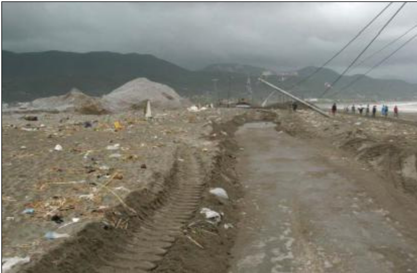
Plate 2: Sediments deposited along the Palisadoes roadway after Hurricane Ivan (2004).
