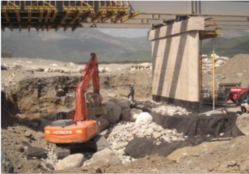
Plate 6: Replacement of the Harbour View Bridge, St. Andrew. The original bridge was severely damaged during tropical storm Gustav. Source: NWA 2010.
