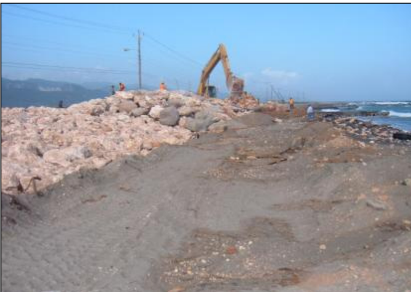
Plate 3: Reinforcement of the Palisadoes roadway.
