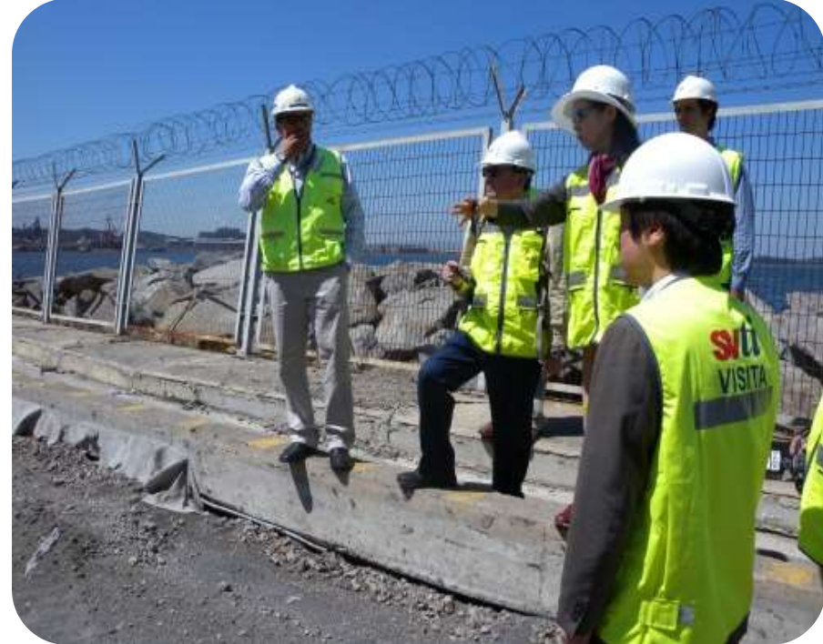
Damage Inspection at Talcahuano, Chile
