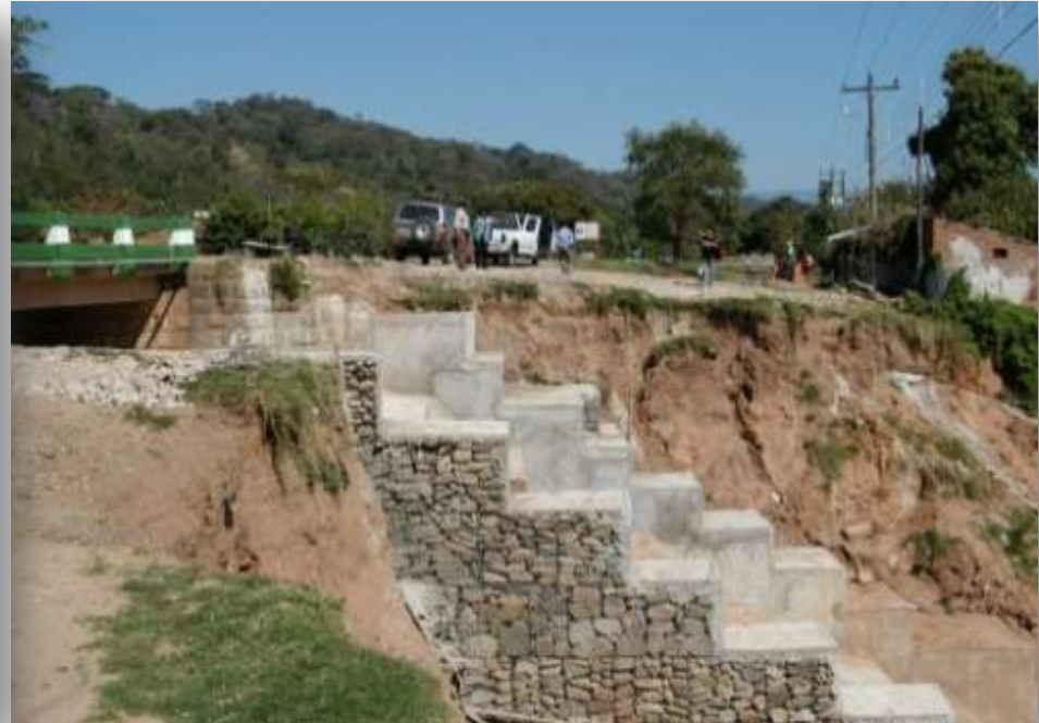
Shoulder protection works at National Road 7 in Bolivia
